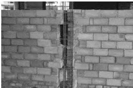
墙体预埋钢筋
