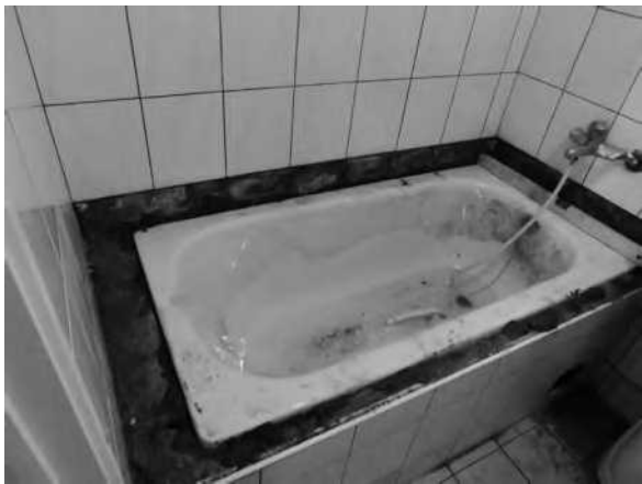
拆除砌筑式浴缸
