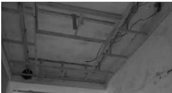
暗藏灯带木龙骨安装
